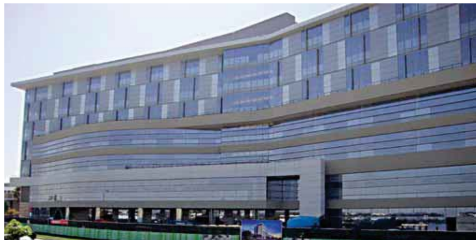
Torrance Memorial's new main tower. Photos by TerriAnn Ferren.
